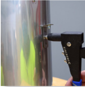
Rivet all four mounting brackets to the termination.
