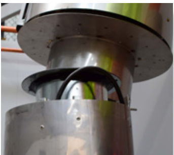
Flip the cable inwards and fit the termination to the roof penetration.
