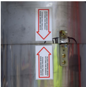
Ensure both the arrows on the termination and penetration are aligned for easy cable fitment.
