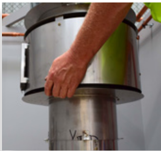
Flip the cable inwards and fit the termination to the roof penetration.
