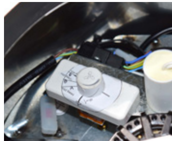
Pull the cable to the top of the termination and attach to the connection block as shown below. Please ensure that the leads do not touch the motor in any way (cable tie if necessary).
