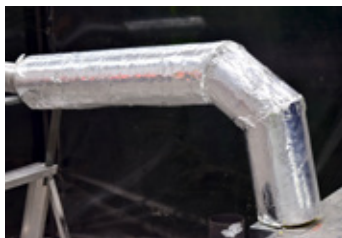
Bends where practical should be insulated, by cutting the insulation into segments and taping together.
