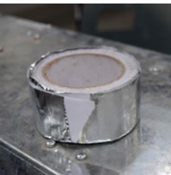
Joins can be taped together using aluminum foil self adhesive tape.
