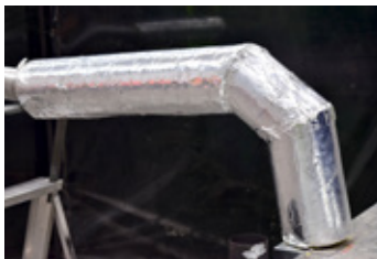
Bends where practical should be insulated, by cutting the insulation into segments and taping together.
