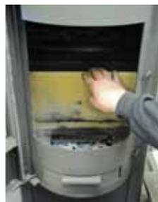
7. Lift the top baffle plate free of the brackets and down and back from the brackets to release it.
