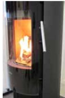
4. When you can see that the chimney is hot enough to draw (after 5-10 minutes), close the door. If all the necessary conditions are met, a thick layer of embers will have been formed in the combustion chamber after another 15-20 minutes.
